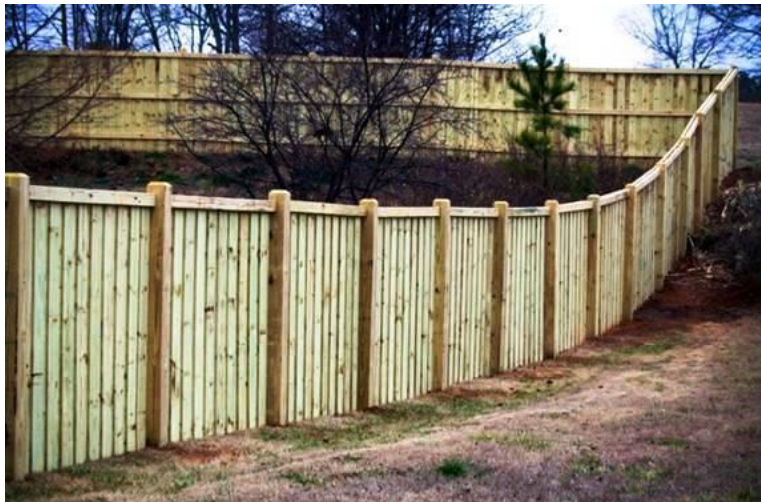
Figure 25-5.5.6: Fence with Finished Side Out
